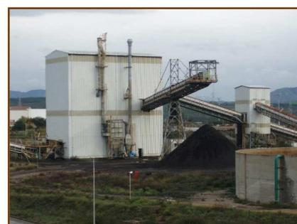
**Floatation:** Plant for the recovery of the thin part of coal as well as of the high value special materials :
