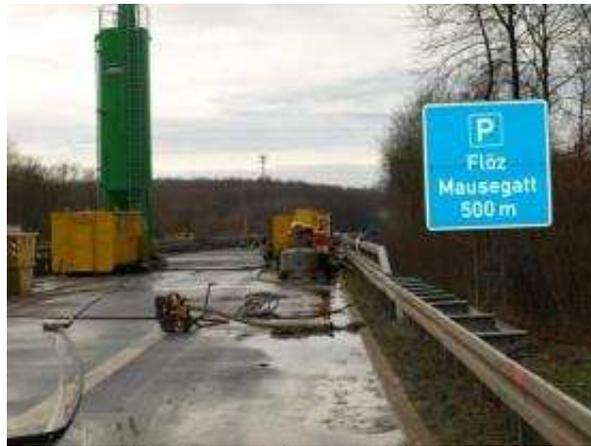
*Figure 1: Remediation of mine subsidence on the German Highway (BAB 45).*
