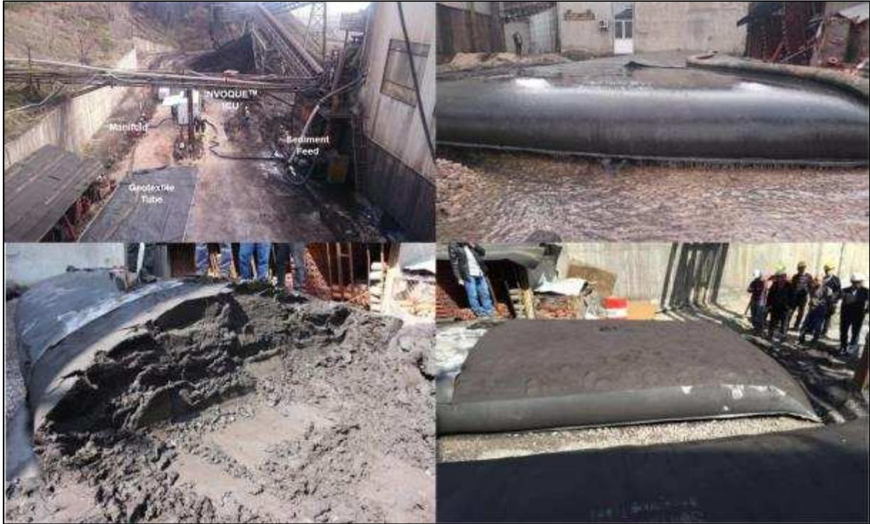
Fig. 4 Clockwise from top-left: staging area, dewatering, opening of tube, during excavation.
